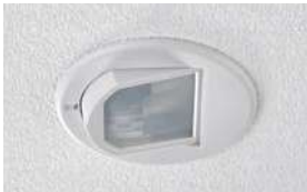
Detection head position set to 15°
