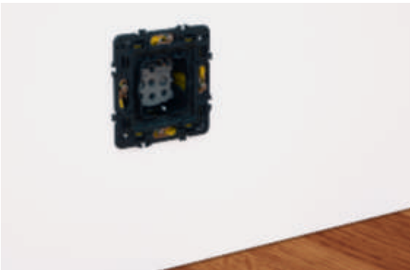
3 Assemble the mechanism in the support
