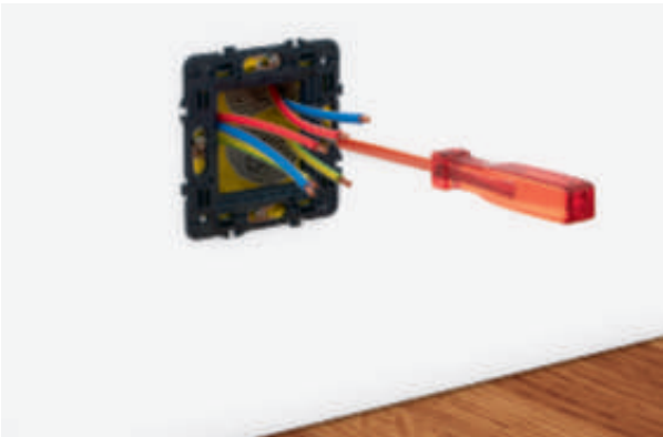
1 Fix the support on the box
